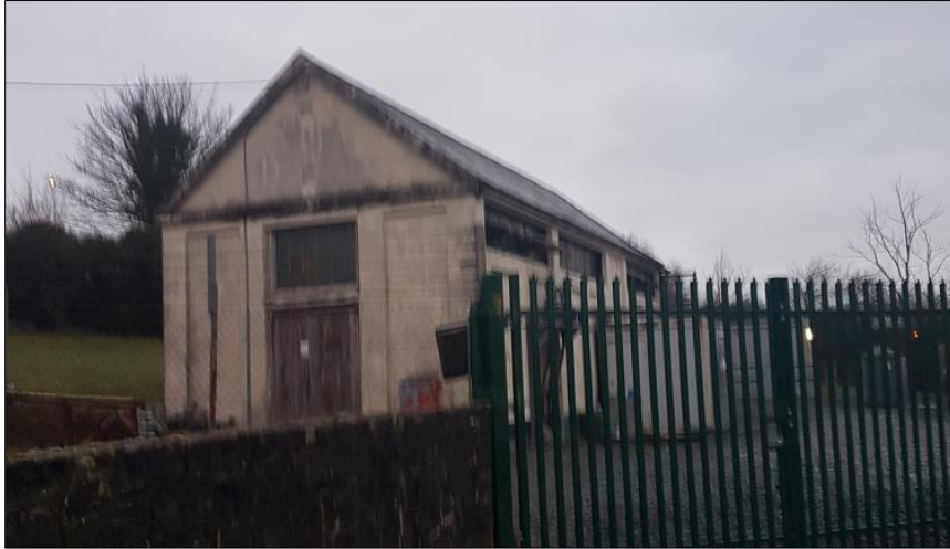
Figure 5. Roadside View of Corrawarrin 38kV site.
